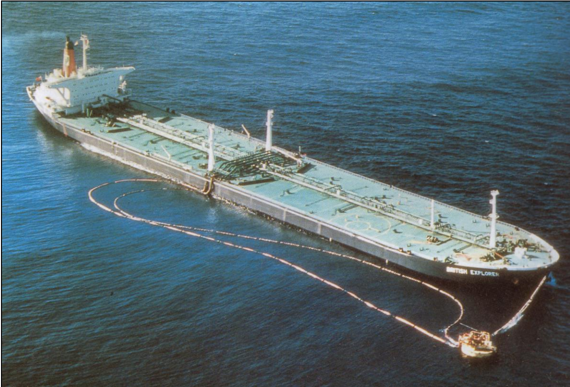
SPM (Single Point Mooring)
